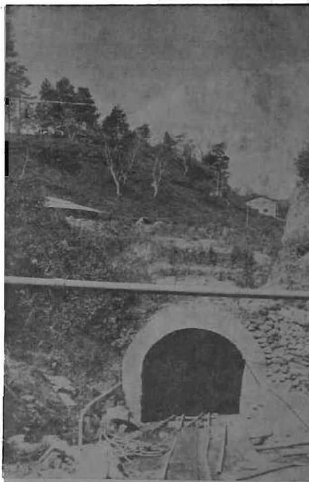
The Tunnel at Pallivasal.
