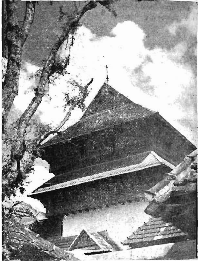
An exterior view of the Chamber of Murals, Padmanabhapuram.
