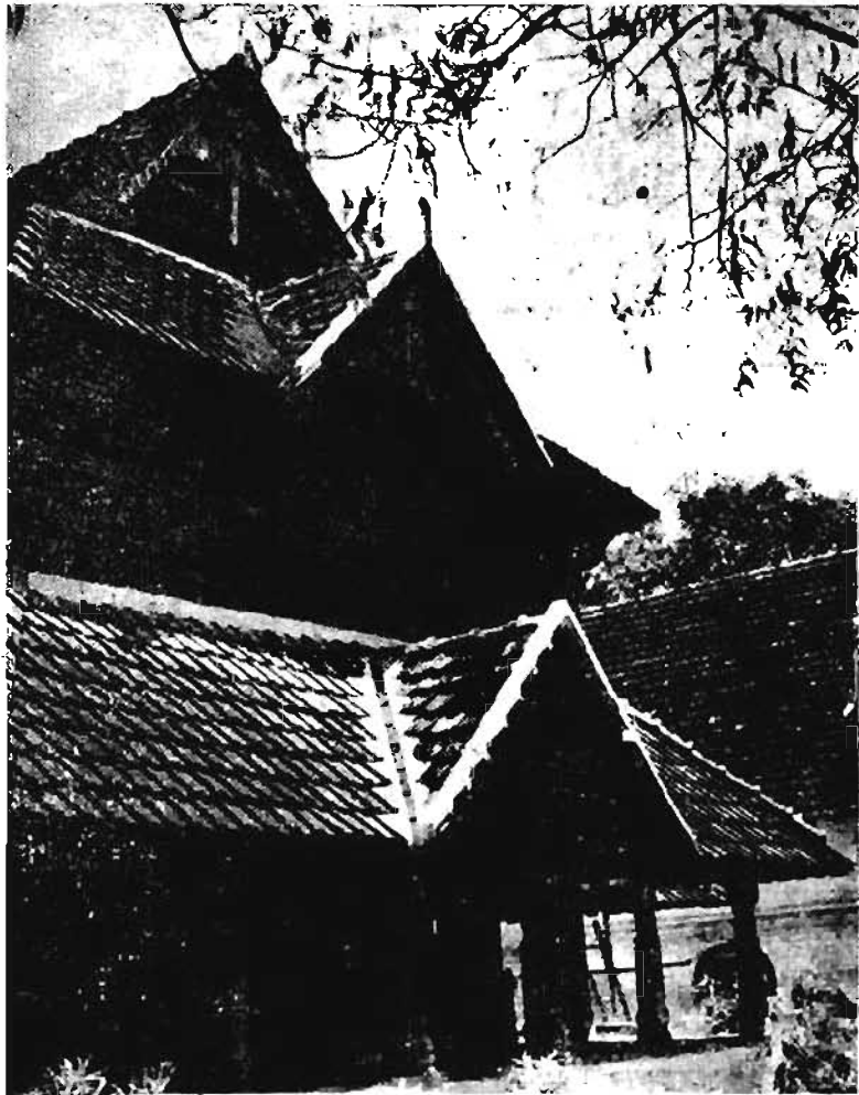
The Entrance to Padmanabhapuram Palace, now a Temple of Art.
